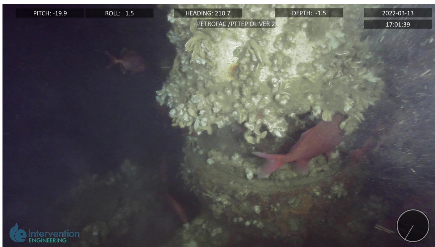
Figure 12 Oliver 2 Example of corrosion on wellhead
