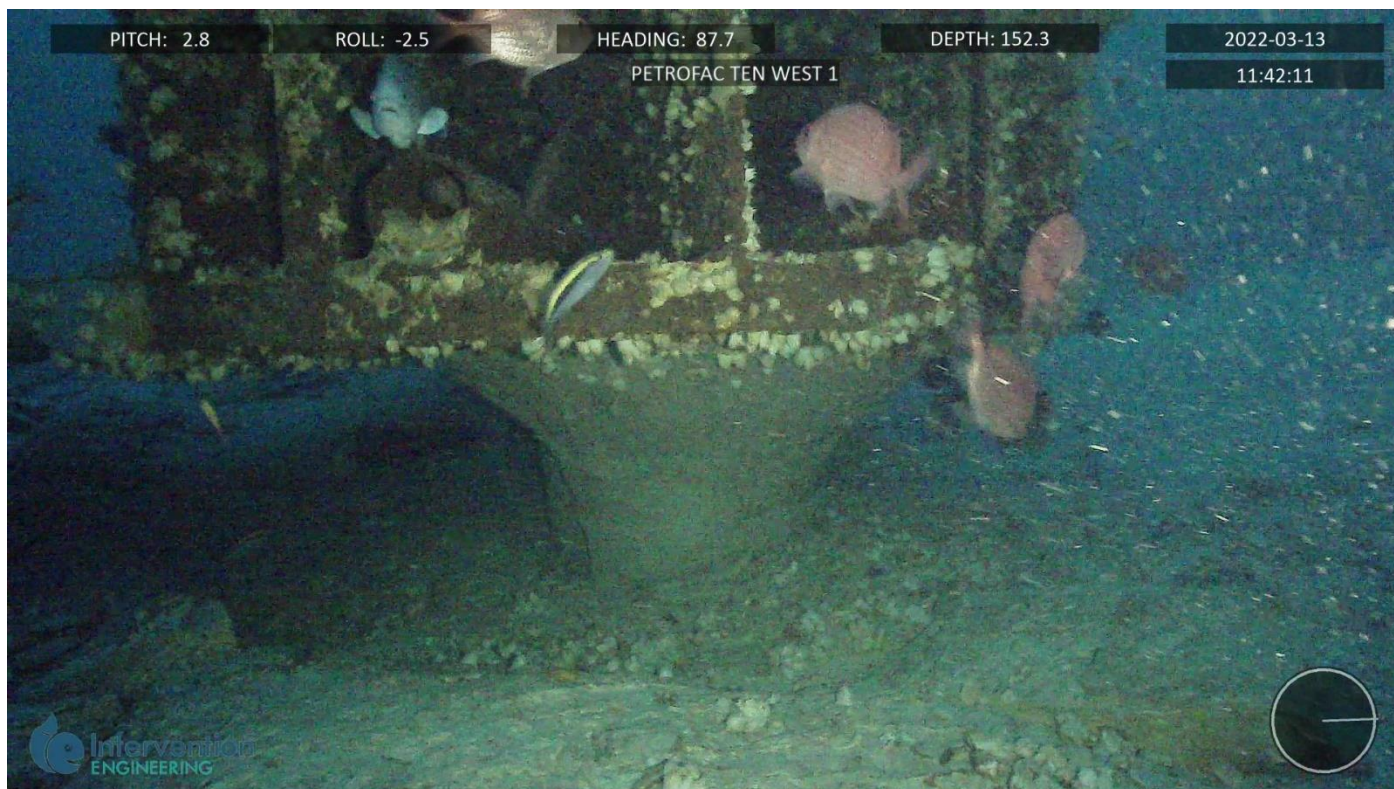
Figure 6 Ten West 1 example scour under guide base
